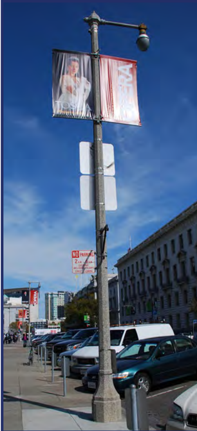
Aggregate concrete streetlight post with right angle pendant on Grove St
