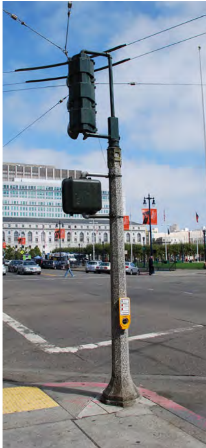
Modified aggregate concrete post with traffic signal
