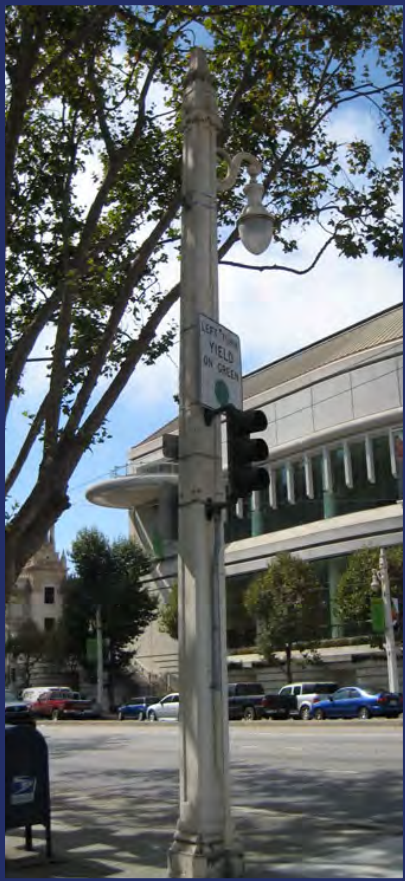
Van Ness trolley pole with single pendant and signal
