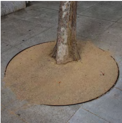
Tree well along Van Ness Ave - circular, metal edging, filled with decomposed granite
