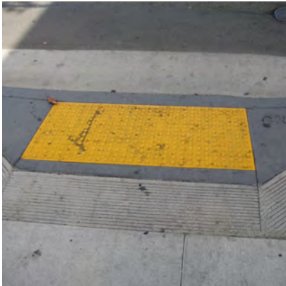
Accessible ramp with truncated domes
