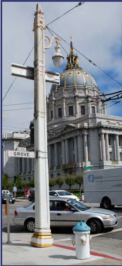
Van Ness trolley pole with single pendant and high pressure auxiliary water supply hydrant
